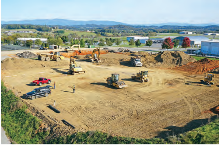
The site of the new Technical Education Complex in late October.
