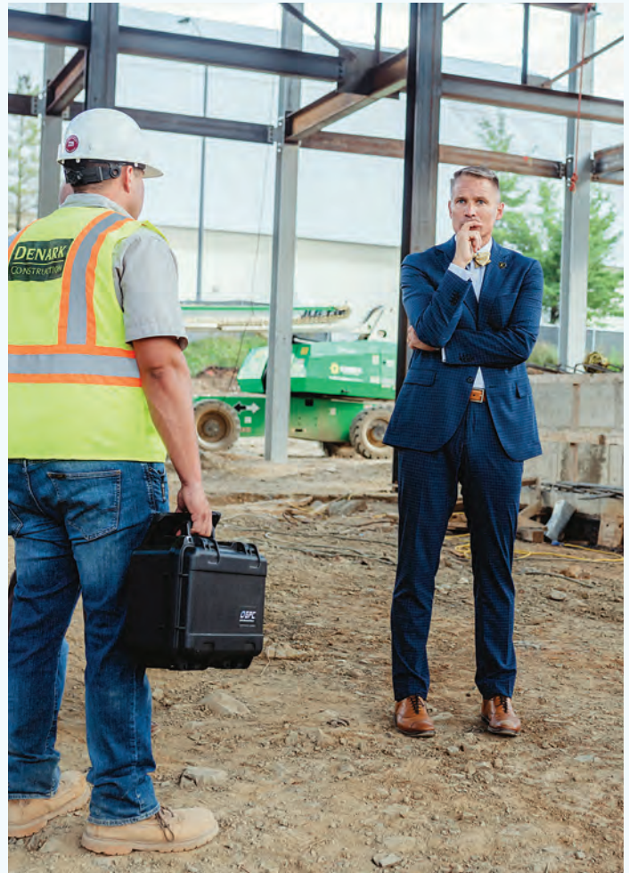
Noland listens to an update on construction of the Martin Center from Abbie Forrest of Denark Construction. PHOTO BY TARA HODGES, SWEET SNAPS PHOTOGRAPHY.
